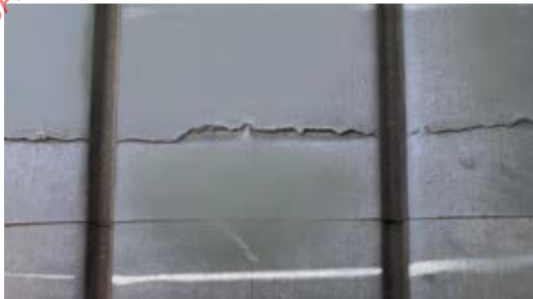
FIGURE 16 - OPEN TREAD SPLICE
