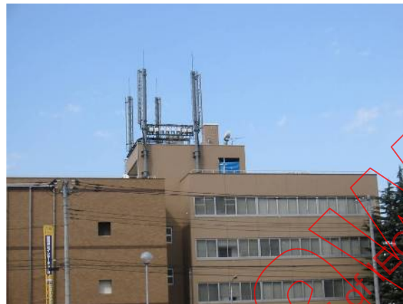
Figure P.5 – Roof-top case study with large antennas and no direct access
