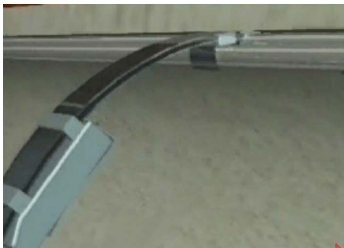
Figure D.2 – Spring loaded stainless-steel ring – conduit fastening
