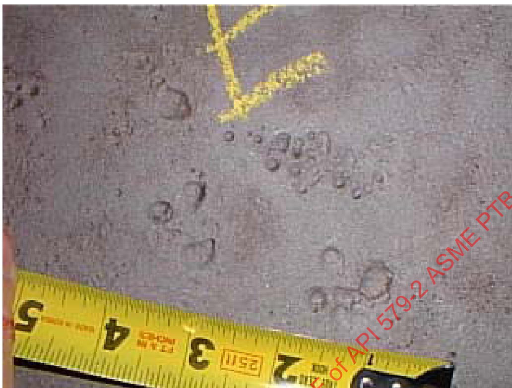
Figure E6.1-1 Example Problem E6.1 Pitting Damage
